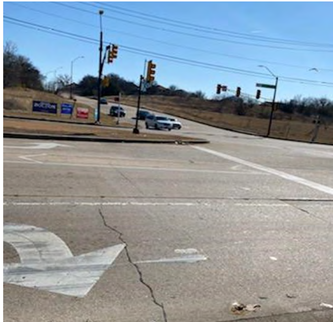
Marked Crosswalks Needed at Intersections
