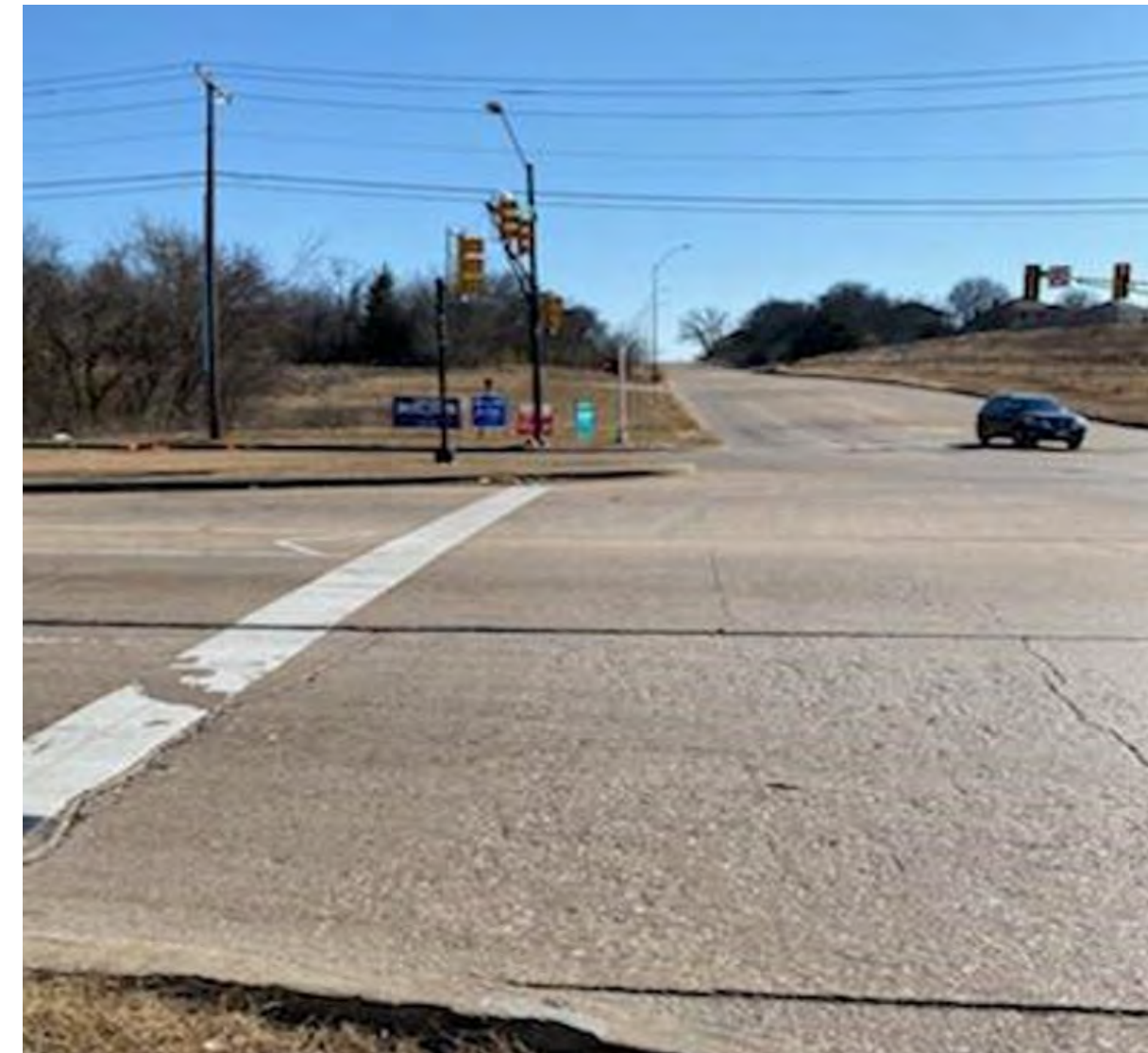
ADA Ramps Needed at Intersections
