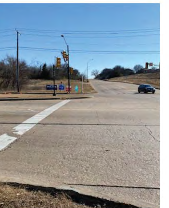
Intersections will need to be made ADA compliance
